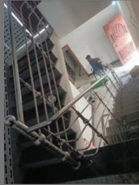
Mild Steel Staircase Railing
