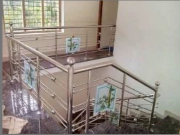
Silver Stainless Steel Staircase Railing
